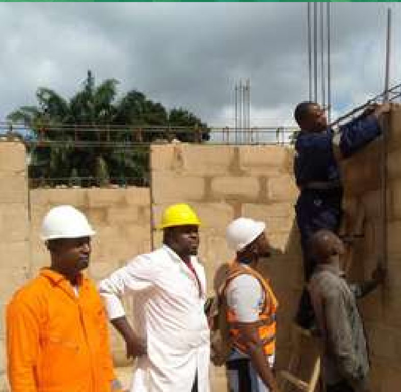
ELECTRICAL TEACHERS WORKING AT THE EUROPEAN BUSINESS PARK
