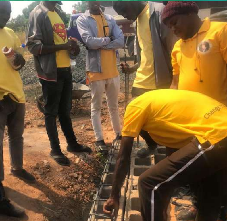
MASONRY FIELD WORK
