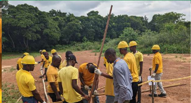
MASONRY FIELD WORK
